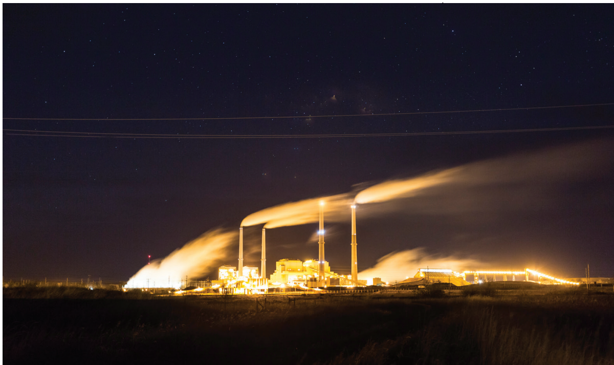
Colstrip Power Plant. Photo by Colin Ruggiero.
