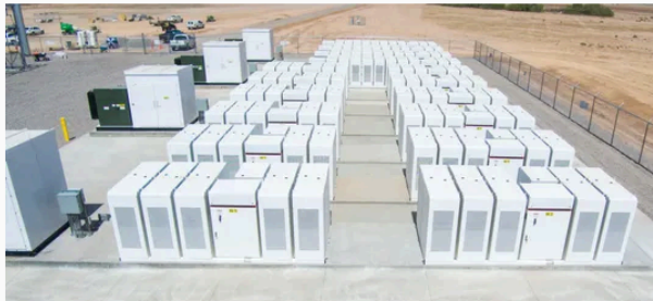
The Pinal Central Solar Energy Center is a 20-megawatt solar plant east of Casa Grande. Salt River Project announced a much larger project Nov. 14, 2019. (Photo: Salt River Project)
