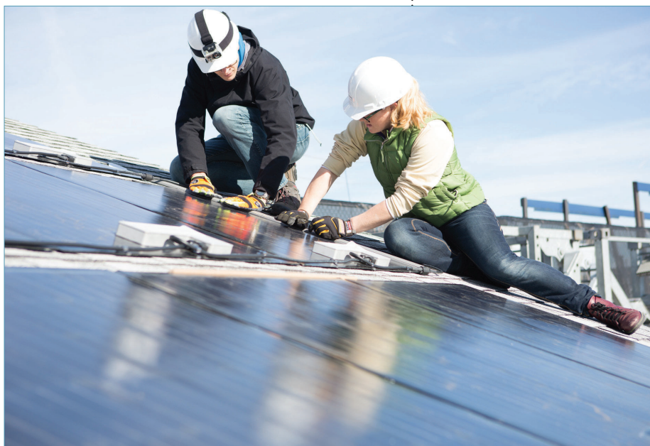
Workers installing solar panels.
