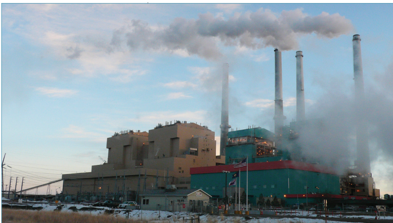
Colstrip Power Plant.
