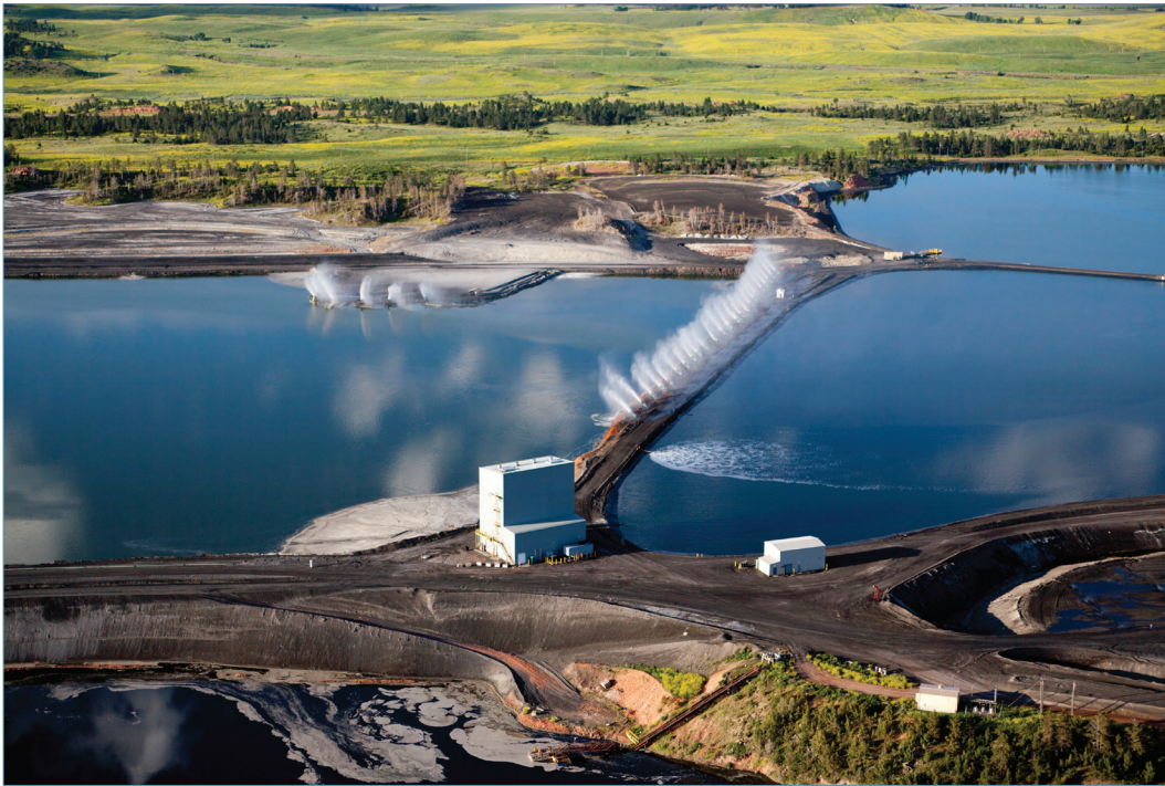
Coal ash ponds at Colstrip Power Plant.
