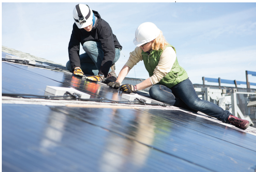
Workers installing rooftop solar panels.
