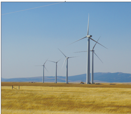
Judith Gap wind farm in Montana.
