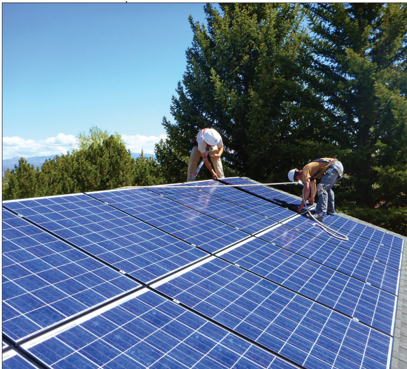
Rooftop solar installers.
