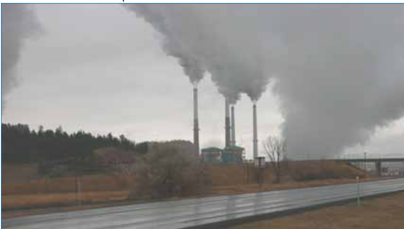
Colstrip coal-fired power plant.
