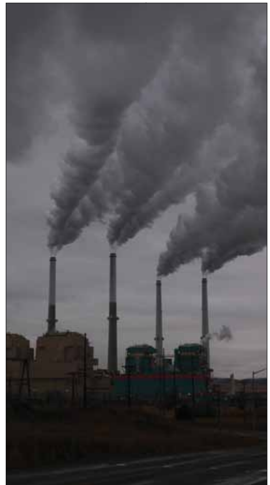
Colstrip coal-fired power plant.
