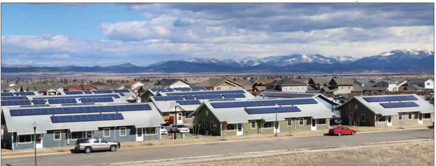
A large solar energy installation in Helena. Photo by Jessica Jones/Solar Montana.
