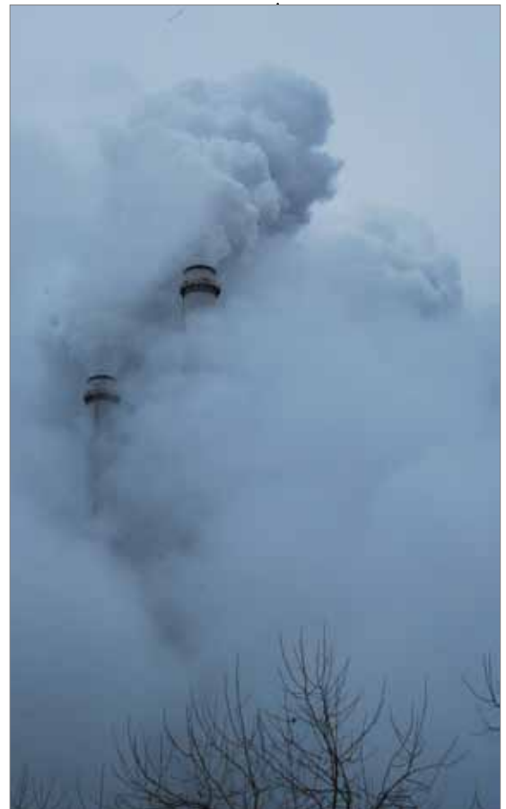
Colstrip coal plant.
