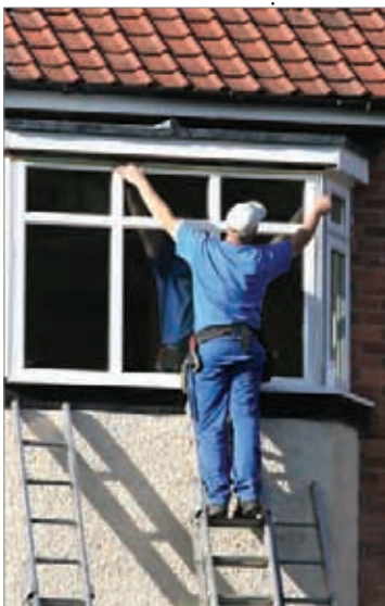
Installing energy efficient windows. Photo by MEIC.
