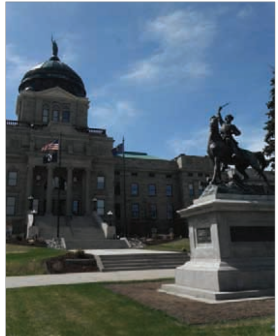
The Montana Capitol building.
