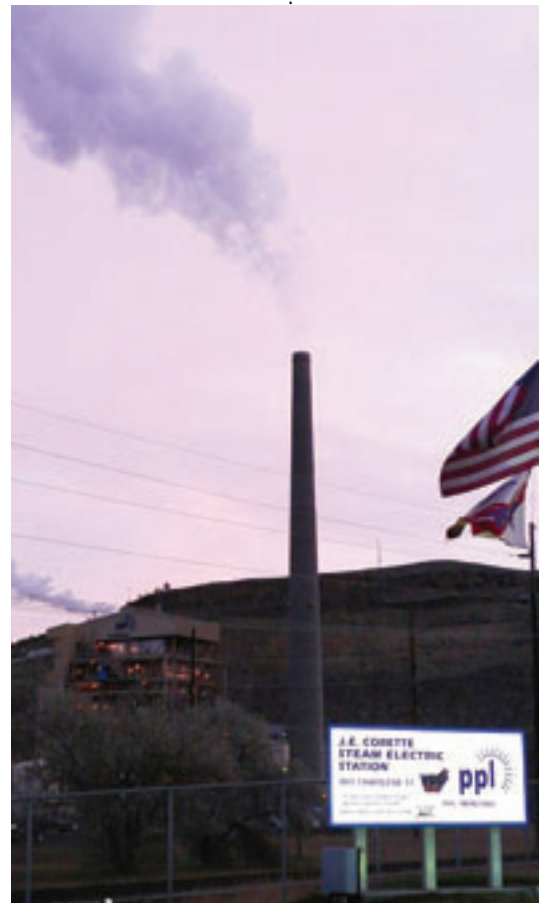
The Corette Power Plant in Billings. Photo by MEIC.
