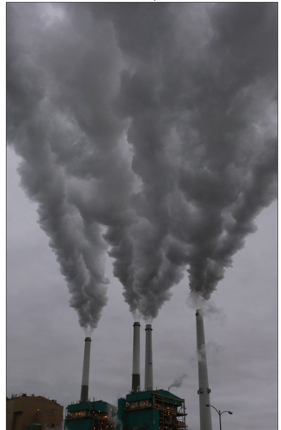
Colstrip Power Plant. Photo by Anne Hedges.
