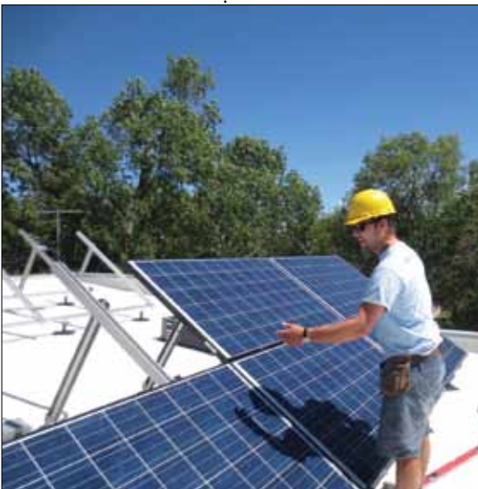
Solar Montana installing panels on a Helena, Montana home.
