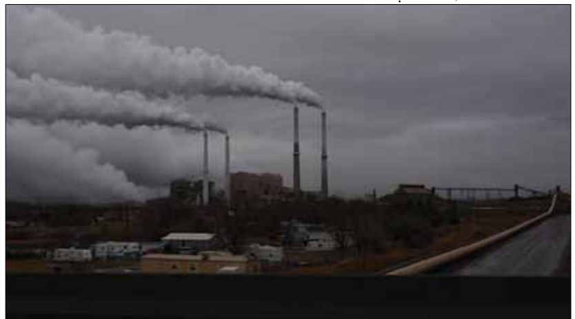
Colstrip Power Plant.
