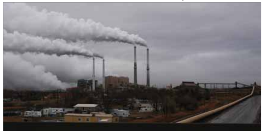
Colstrip power plant. Photo by MEIC.
