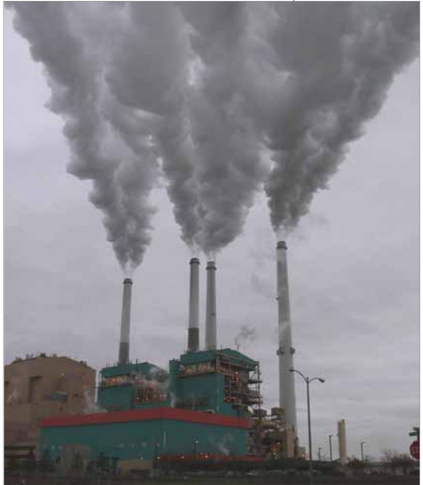
Colstrip coal-fired power plant.
