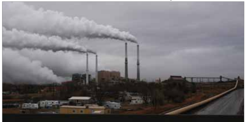
Colstrip power plant. Photo by MEIC.
