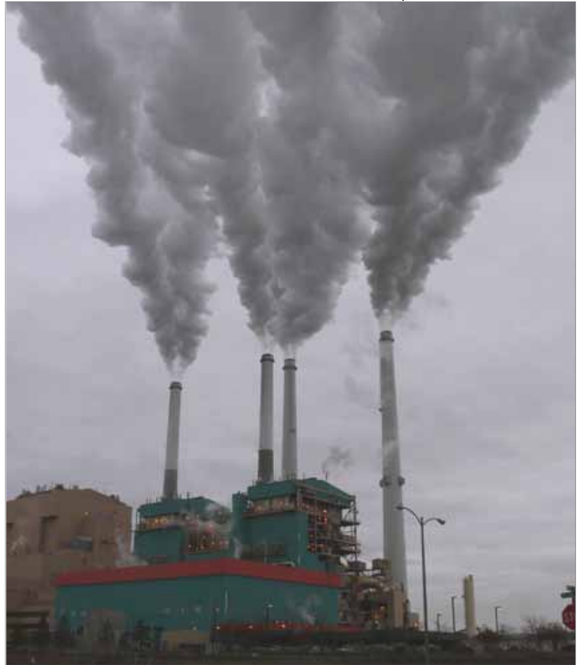
Colstrip coal-fired power plant.
