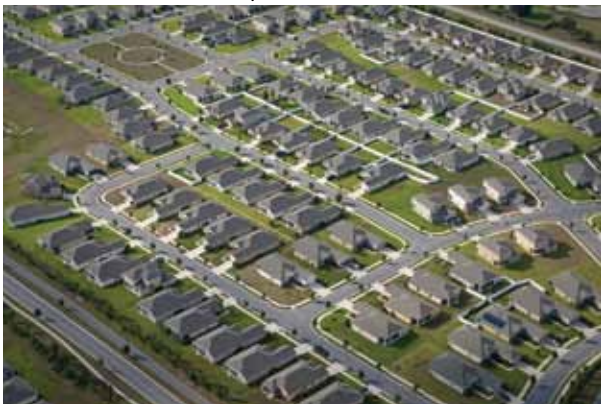
Sprawl from poor land-use planning.
