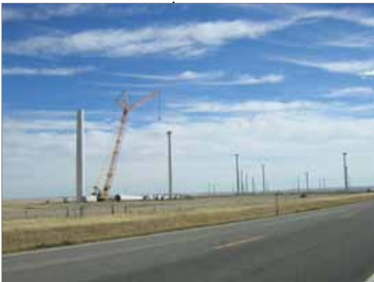
Construction of the Judith Gap Wind Farm. Photo by MEIC.
