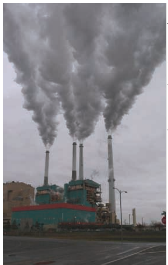
Colstrip coal-fired power plant. Photo by MEIC.
