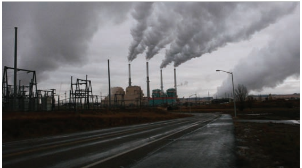
Colstrip power plant. Photo by Anne Hedges.
