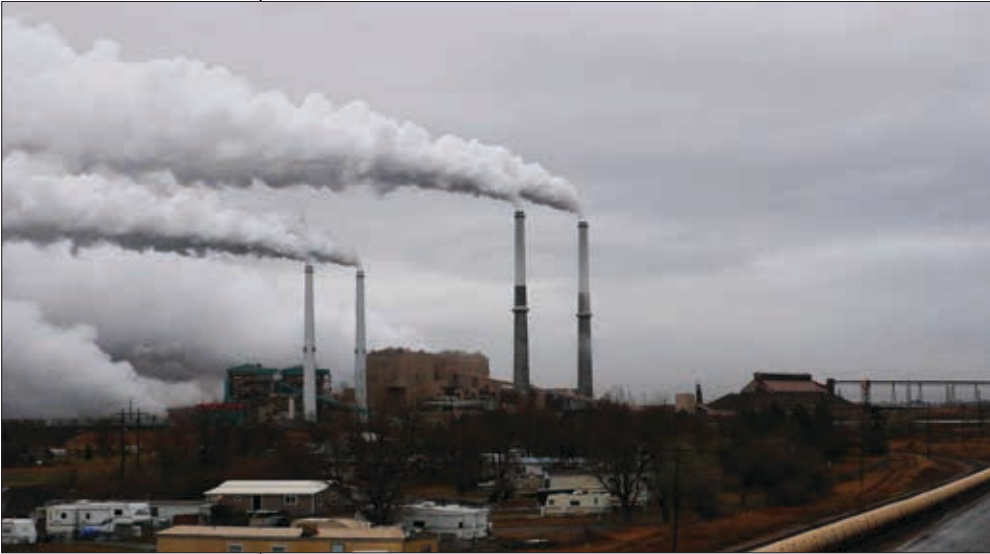
Colstrip Power Plant. Photo by Anne Hedges.
