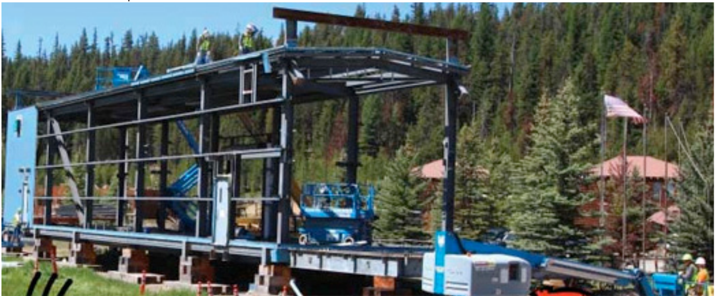
A crew dismantling Imperial Oil's test mega-load vehicle near Lolo Pass. Photo by Steve Seninger of Missoula.
