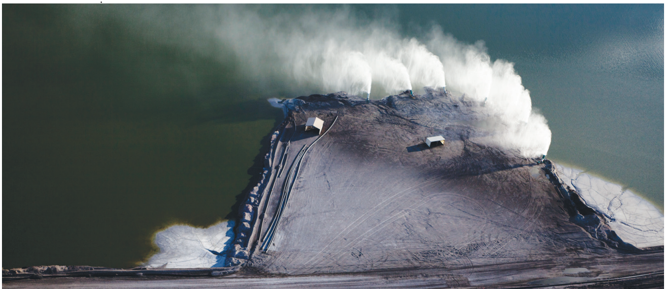
Ash ponds serving the Colstrip facility. Photo by Kestrel Aerial Images.
