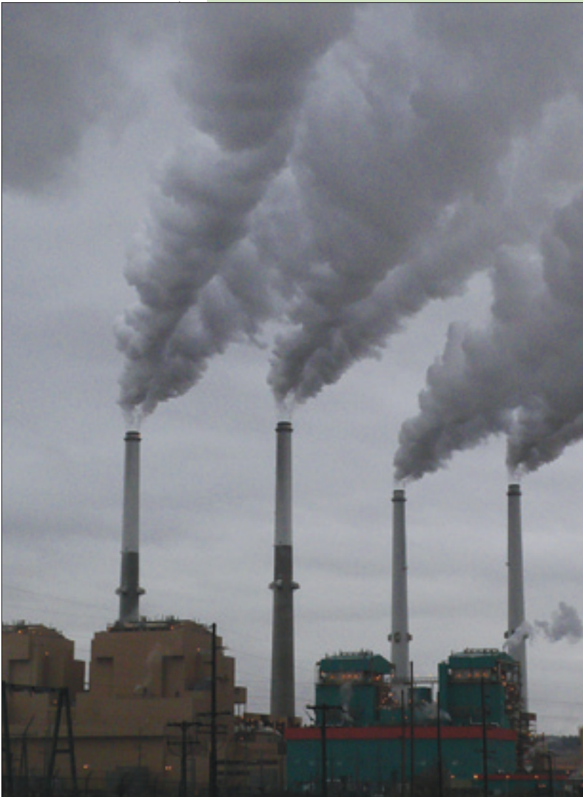
Colstrip power plant. Photo by Anne Hedges.
